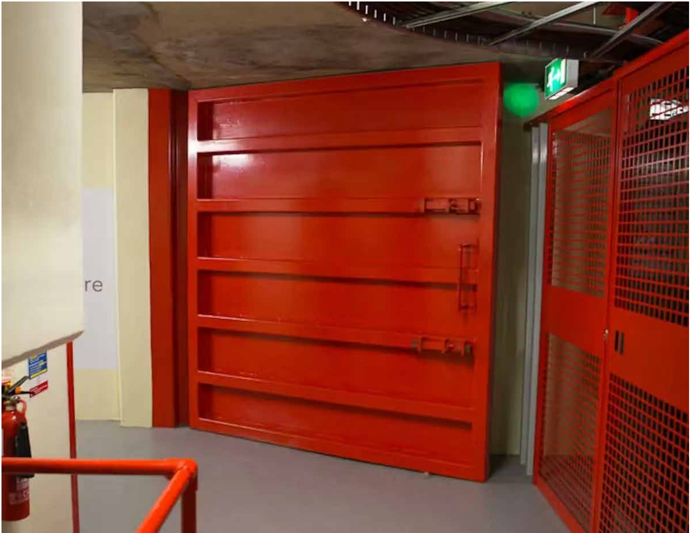
Another heavy duty blast door. PHOTOGRAPH: CYBERFORT/A.R.E. TAYLOR, CC BY
